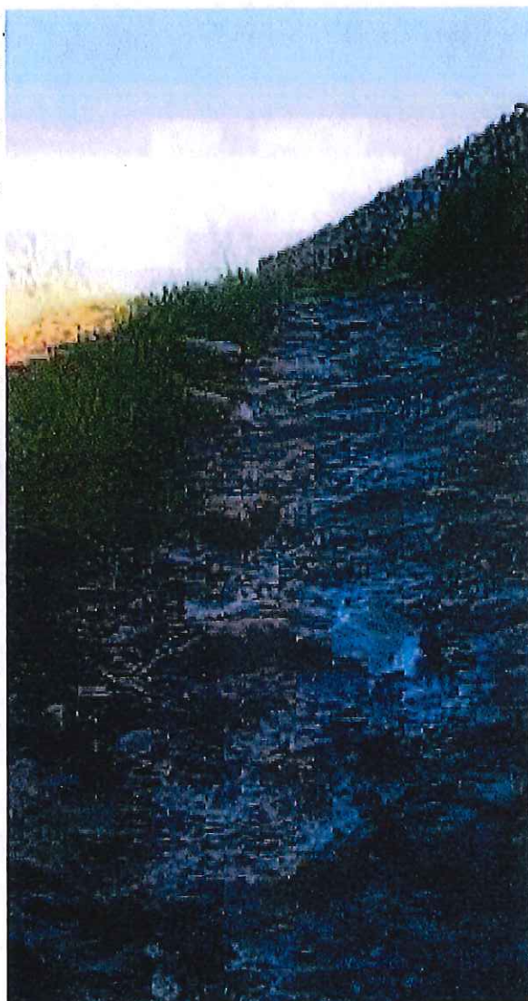
Surface erosion of a route on a gradient
