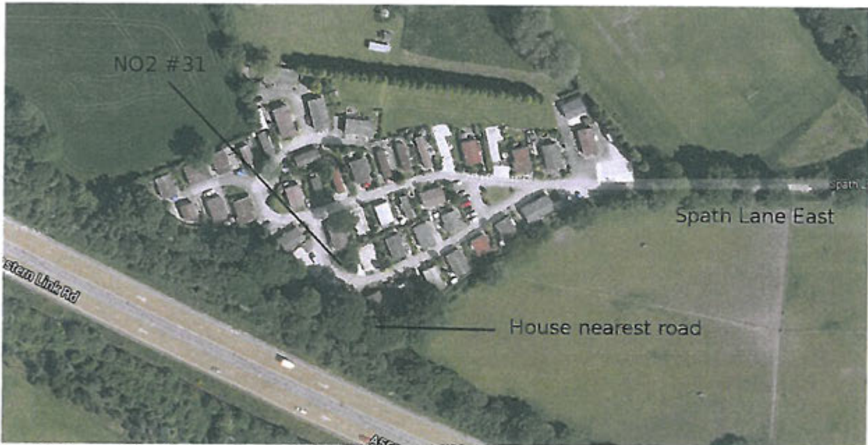
Aerial View of Spath Lane East, A555 in foreground
