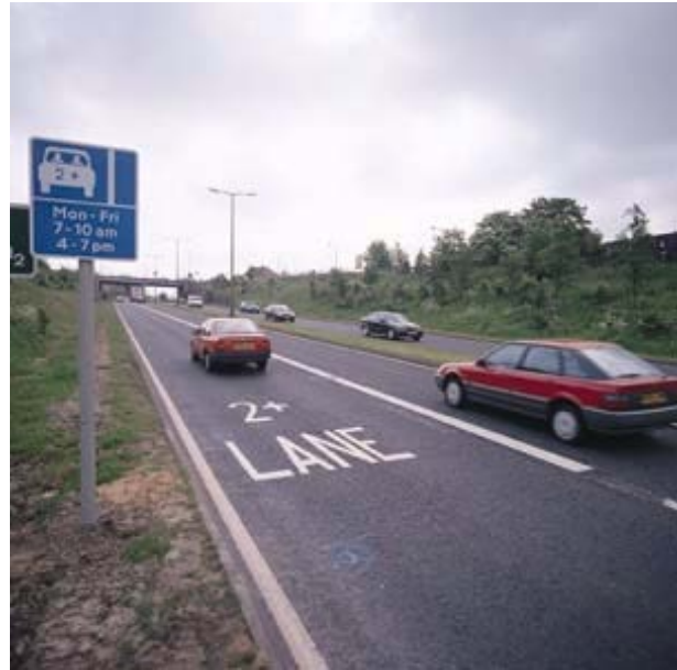
Making better use of local roads: vehicles carrying more than one person benefit from this priority lane in Leeds
