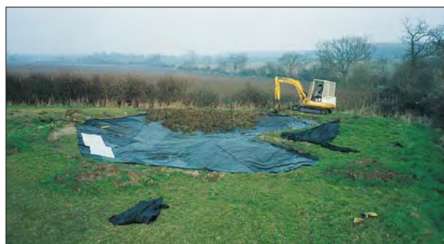
The butyl is put in place, and a further layer of protective matting (polyester) is placed on top. Topsoil is then spread over the pond base to a depth of 50-100mm
