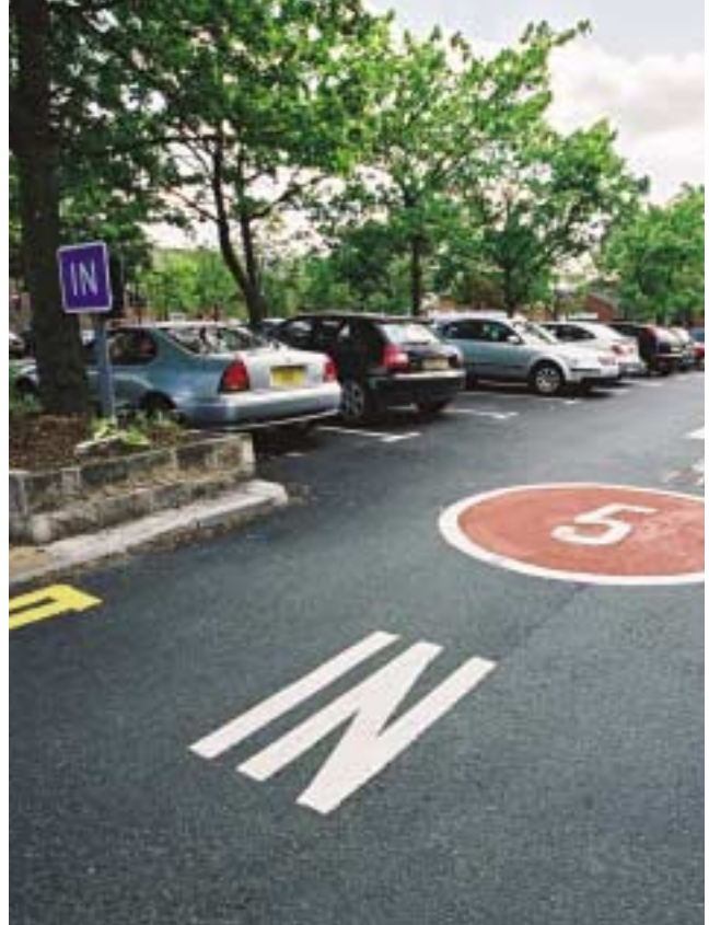
Above: Car park improvements in Cheadle.
