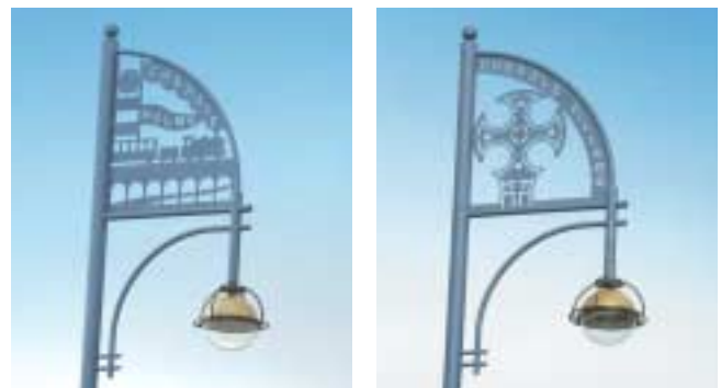
Above: Street lighting improvements.
