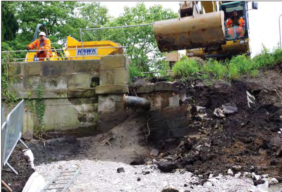
Plate 53: Area 14 Norbury Bridge south wing 14226 being demolished
