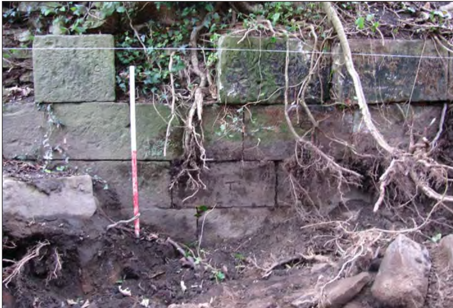
Plate 28: Area 19 head race northern wall 19008, showing masons' marks
