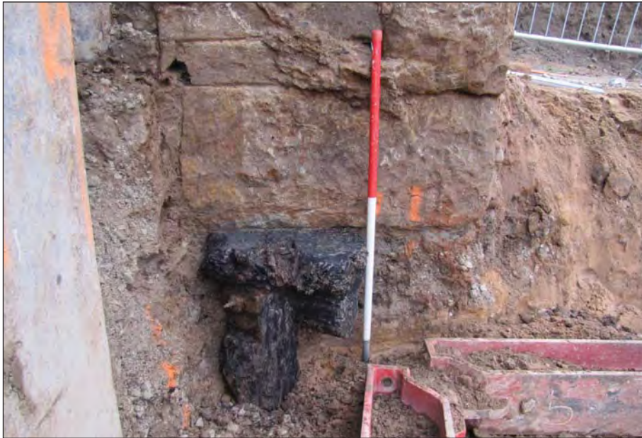
Plate 55: Area 14 Norbury Bridge north side, showing wooden sub structure 14229
