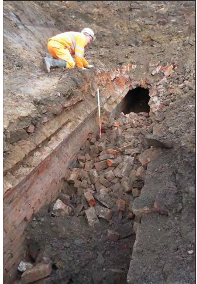
Plate 24: Area 19 tailrace culvert during demolition
