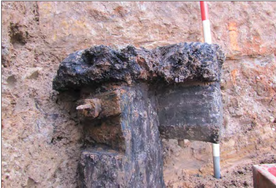
Plate 56: Area 14 Norbury Bridge north side, close up of wooden sub structure 14229
