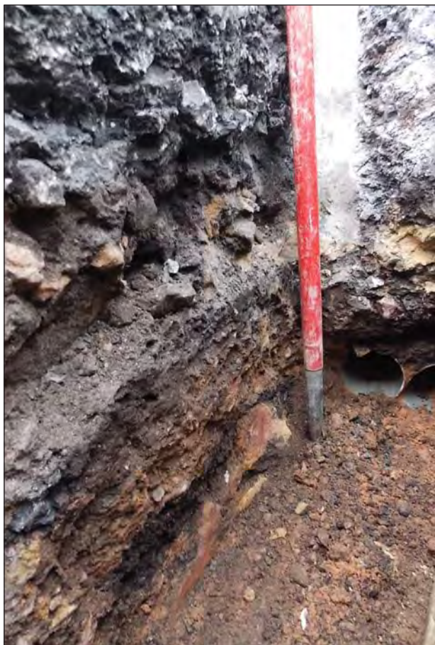
Plate 5: Trench 21.7 cut along the middle of A6, showing possible earlier road surface 21032
