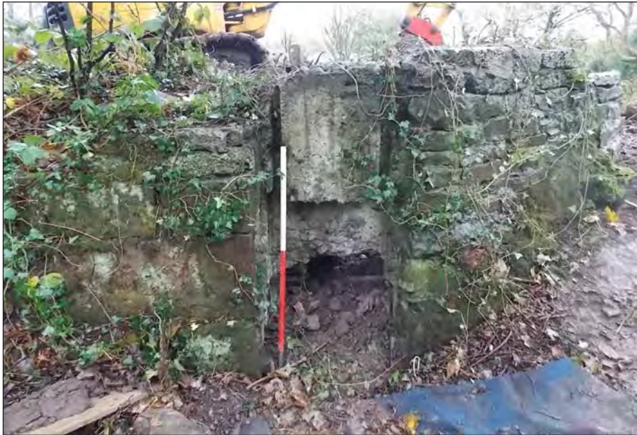
Plate 29: Area 19 head race southern wall 19009, with sluice gate inset 19010
