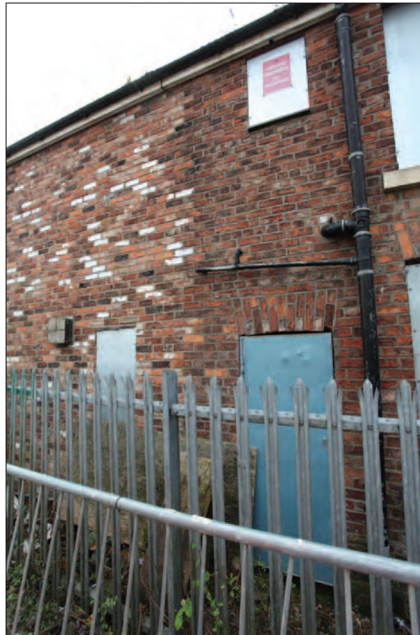
Plate 3: Eastern end of the north elevation of number 83, with vertical construction joint
