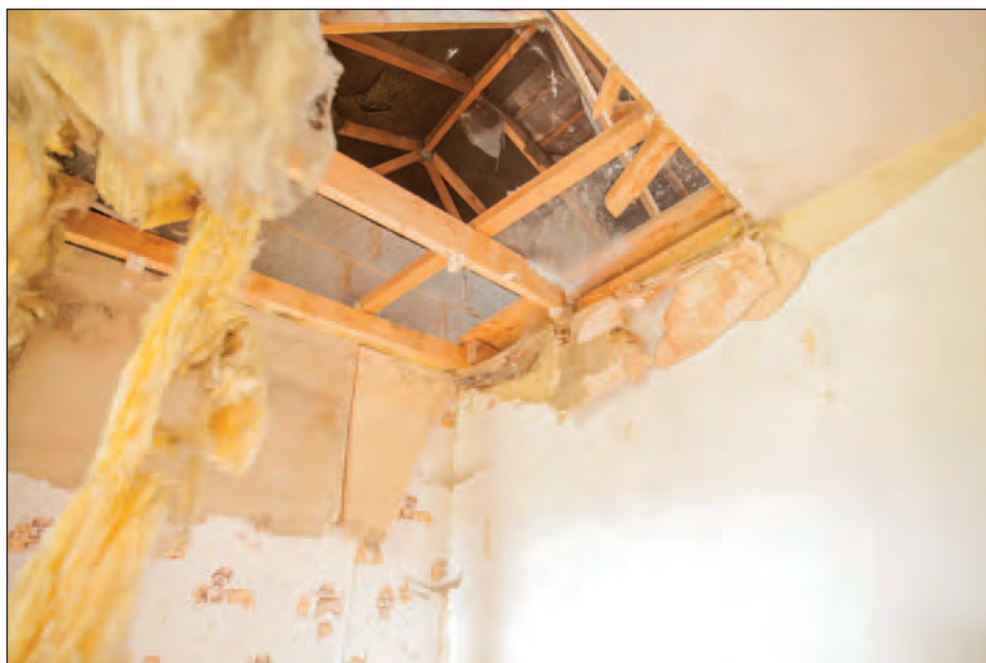
Plate 18: Number 83, room F5 with damaged ceiling showing the roof structure
